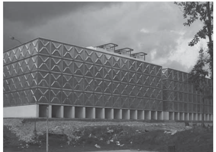
Steel Water Storage Tanks
