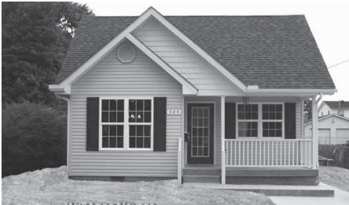
Pre-fabricate steel houses
